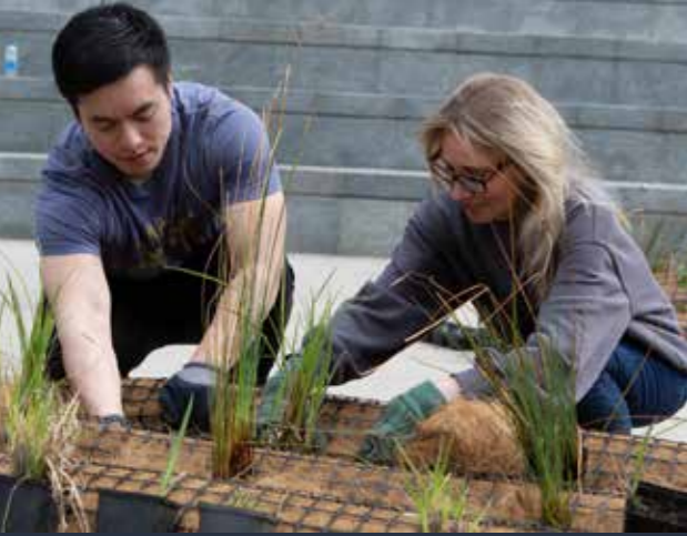
Reed Bed Installations
